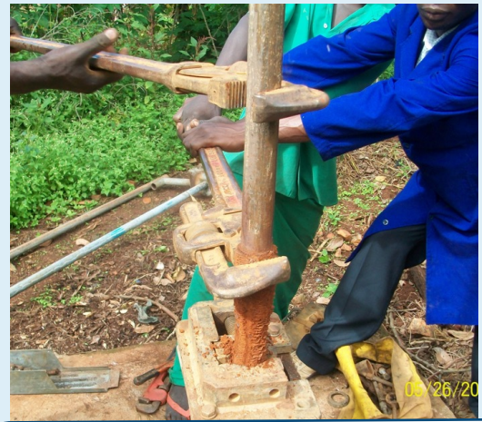
REMOVAL OF A CORRODED WATERWELL RISER PIPE IN HOLMA DISTRICT, UGANDA (source: Larry Bentley)
